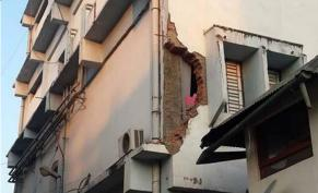
Figure 2.2-1: Damaged properties in Imphal by Earthquake (2016)
