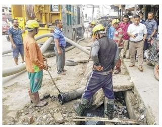
Figure 3.3-2: Repairing of Drain
